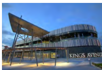
2 KINGS AVENUE MALL
